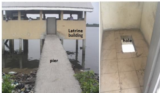
Fig. 1a: Pier Latrine constructed with concrete
